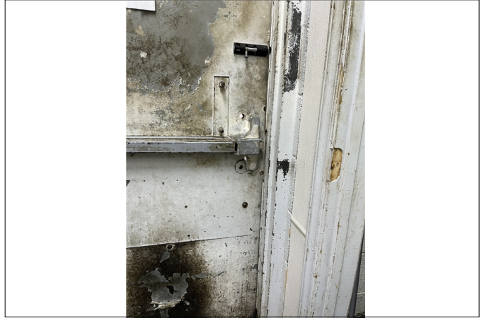
door at cook line
